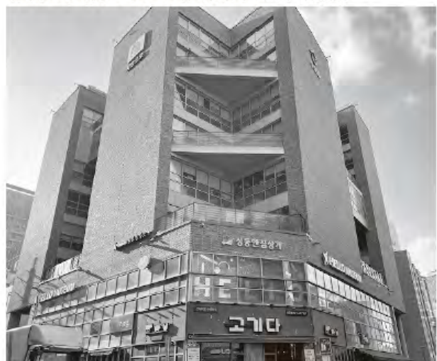
Photo Photo 4: Seongdong Community Assurance Shopping Street Building (photographed in January 2025)
